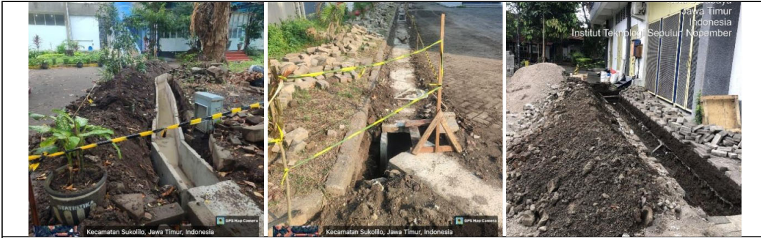
19 Juni 2024 – U-Ditch on site
