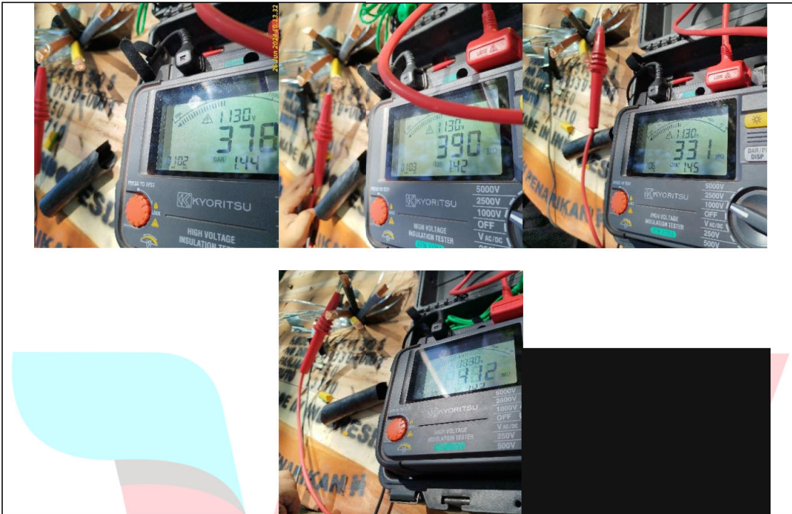
26 Juni 2024 - Insulation test Phase to Ground kabel 185mm sebelum dilakukan pulling
